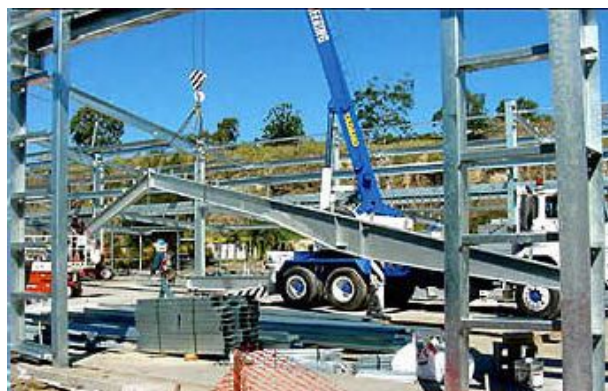
Pierce Engineering: Steel Fabrication and Erection
