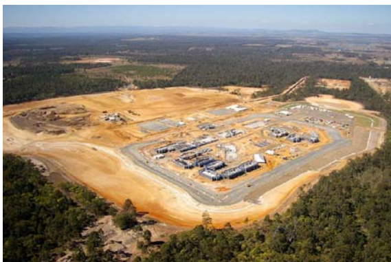
South Queensland Correctional Precinct, Stage 1 source: http://www.uni-span.com.au/images/projects/gatton2.jpg
