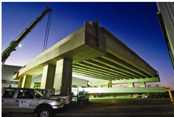
The Gateway project in progress
