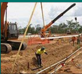
Work on the pipeline
